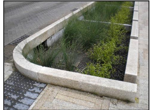
Fig. 3-27-BB: LID stormwater management feature
